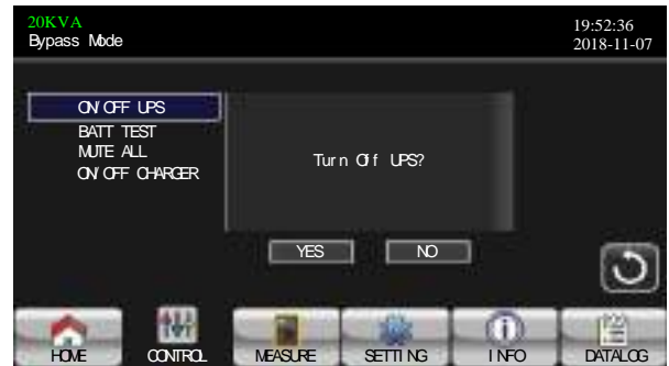
TURN OFF UPS
