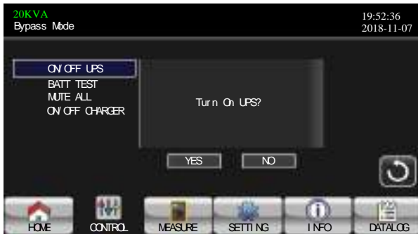
TURN ON UPS
